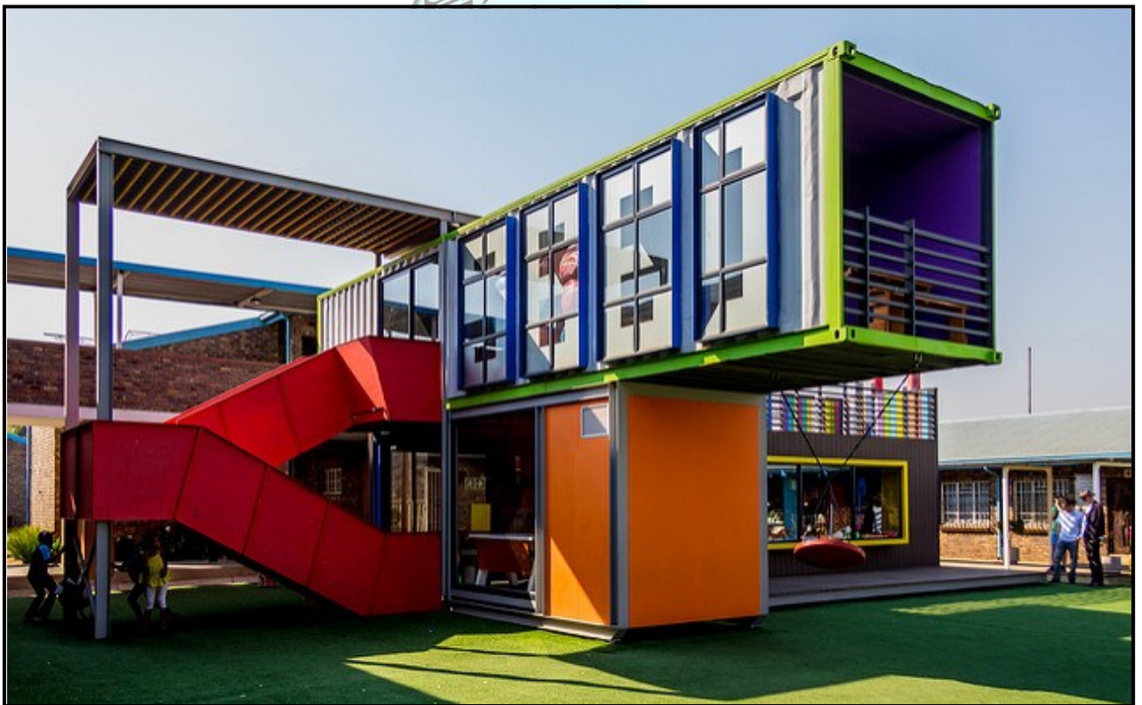
FIGURE 8b: Architects Of Justice, SEED Library II , in Alexandra township, Johannesburg, South Africa, 2010.
