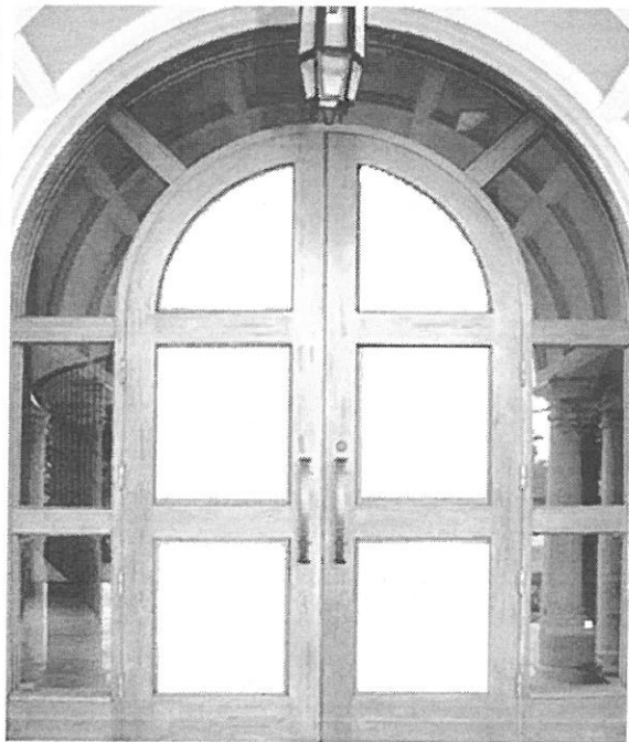
Photograph of the doorway
