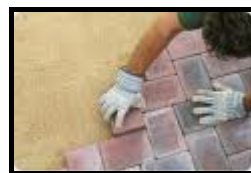
A worker paving the driveway
