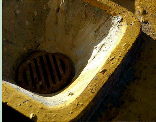
Drains and pipes.
