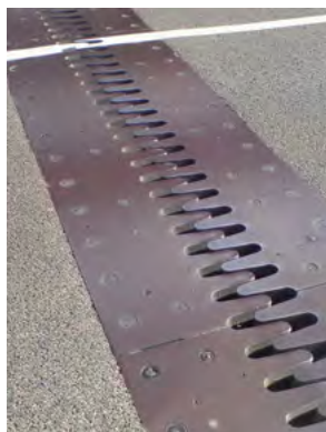
The expansion joint in a bridge.
