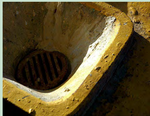
Drains and pipes.
