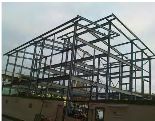
A building under construction. You can see the framework made of steel.
