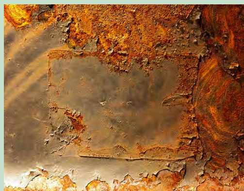
A closeup photo of a rusted barrel.
