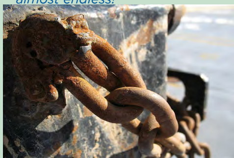
A rusted chain.
