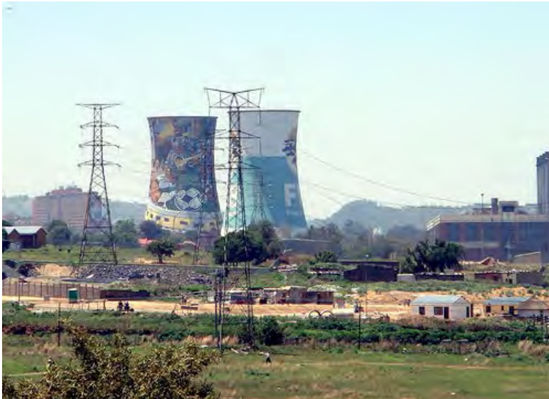
This is the Orlando Power Station in Soweto, which served Johannesburg for 50 years from 1951. It is not used anymore. The painted cooling towers are seen the most prominently, but the building to the right is also part of the power station.
