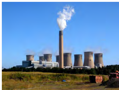
A coal-powered power station.
