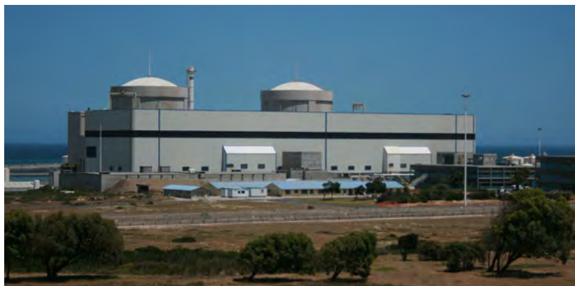
The Koeberg Nuclear Power Station outside Cape Town.
