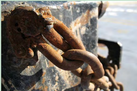
A rusted chain.
