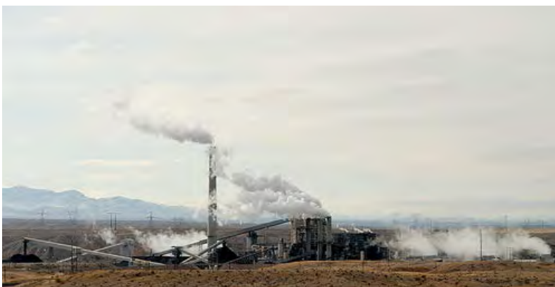
A coal-powered power station.
