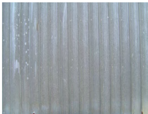
Galvanised panels used for walls or roofs.
