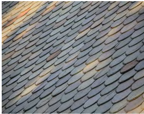
Roof tiles made from slate, which was formed from shale (a sedimentary rock).
