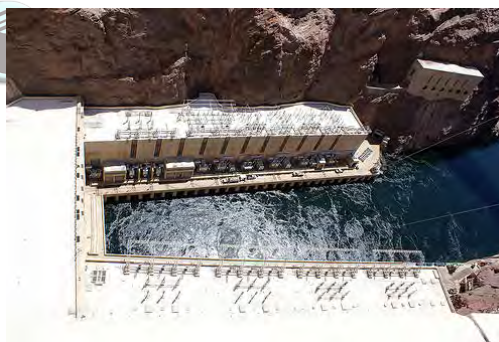
The water then flows out the bottom of the power station and continues down the river.
